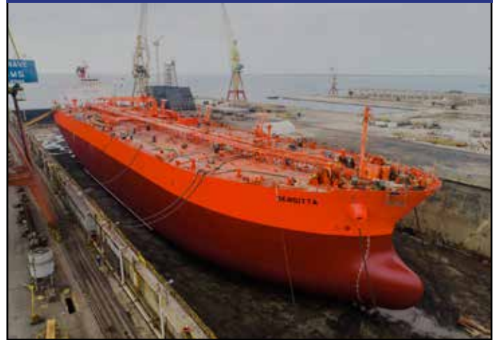
The main graving dock at Lisnave
